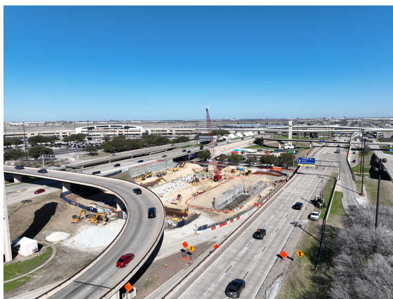
Aerial View of Construction - February 22, 2024
