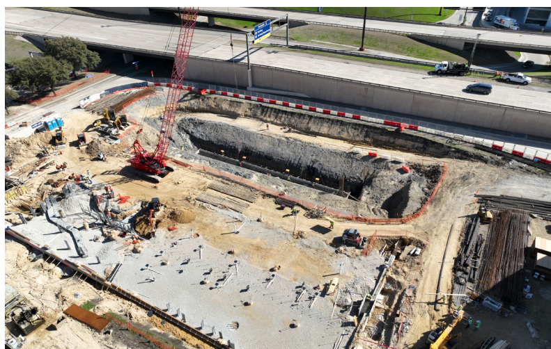
Aerial View of Construction - February 22, 2024
