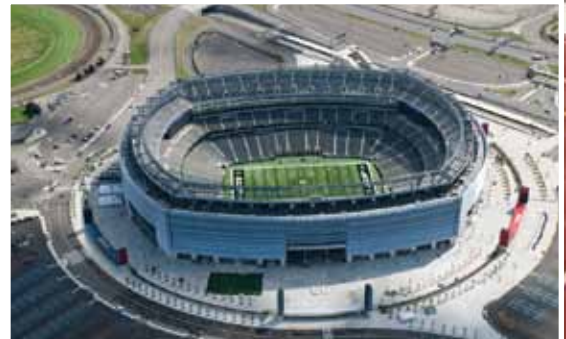
Skanska USA Building Inc. New Meadowlands Stadium East Rutherford, New Jersey
