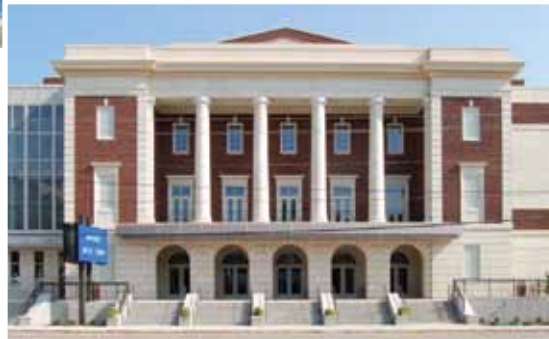
Background photo: MBP/AECOM Joint Venture Washington-Lee High School Arlington, Virginia
