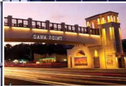
City of Dana Point/PBS&J/TWNiemann, Inc. Pacific Coast Highway Congestion Relief Project Dana Point, California
