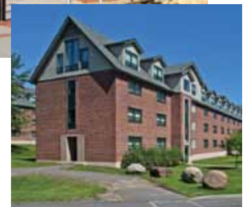
U.W. Marx, Inc. Clarkston University Quad Dorm Expansion Project Potsdam, New York
